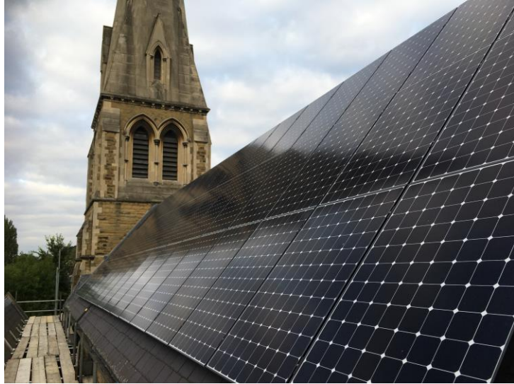
Solar panels and storage (easier for non-listed buildings)
